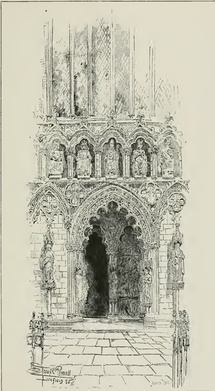
THE CENTRAL DOORWAY, WEST FRONT.
